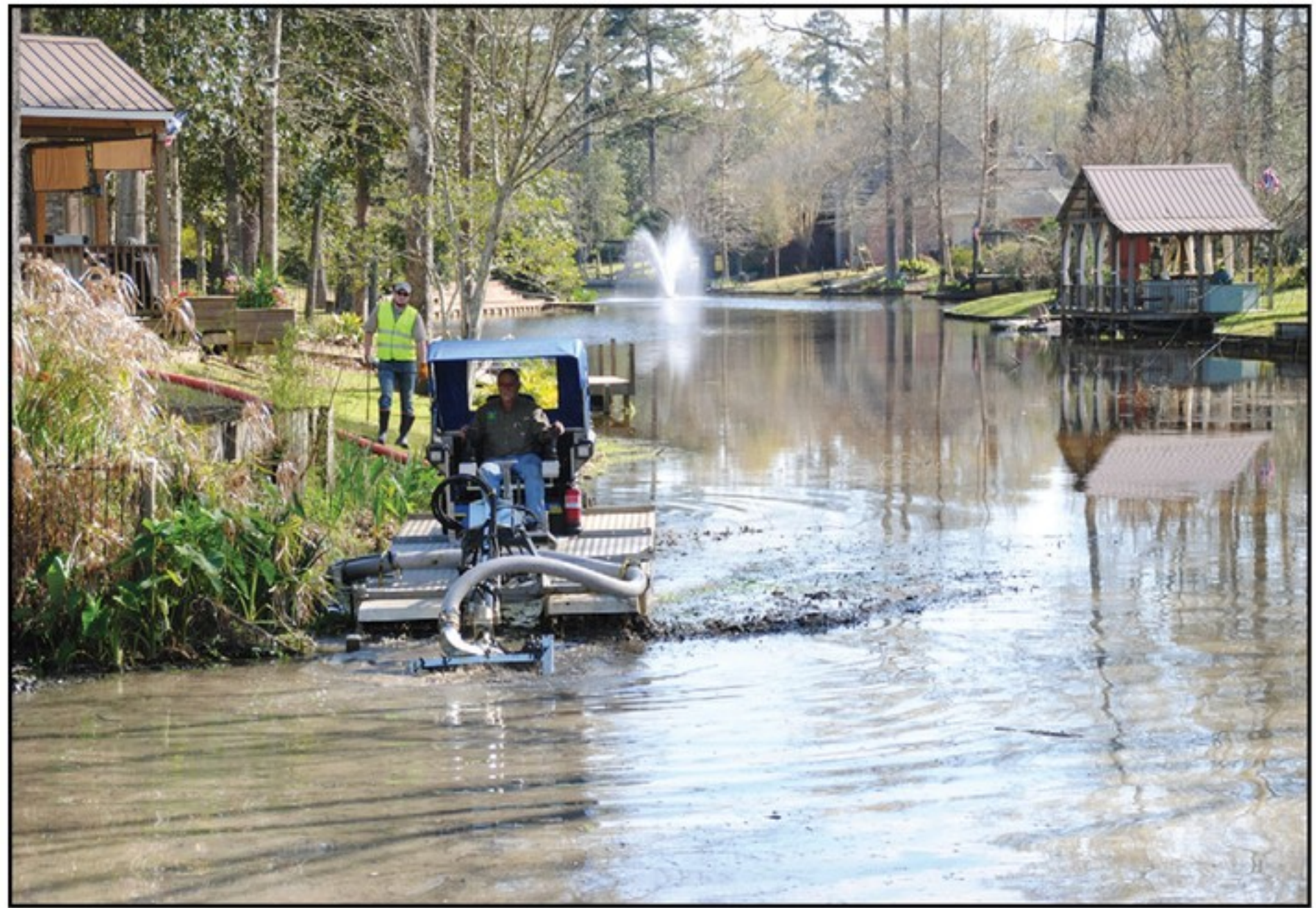
Amphibious dredge running on top of accumulated sediment.
